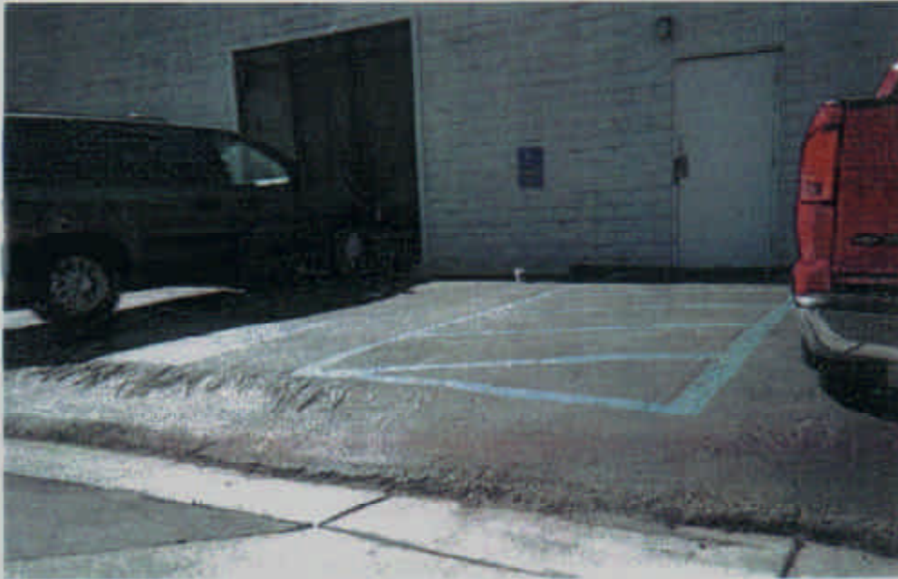
Figure 3 - Narrow space between vehicle and wall. ADA rules require three feet (11/27/01).
