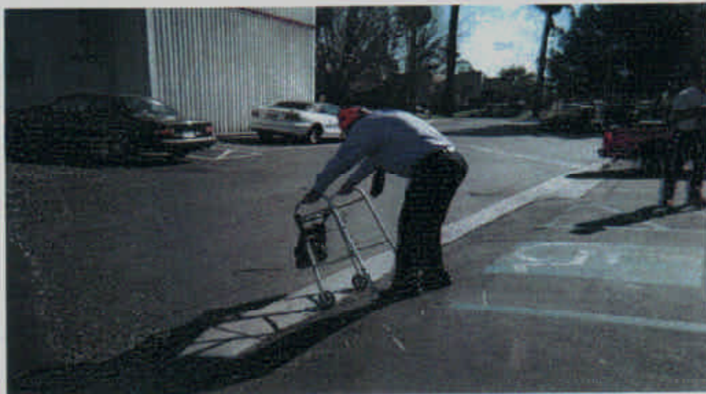
Figure 2 - Difficulty in using a walker or a wheelchair on steep slope (11/27/01)
