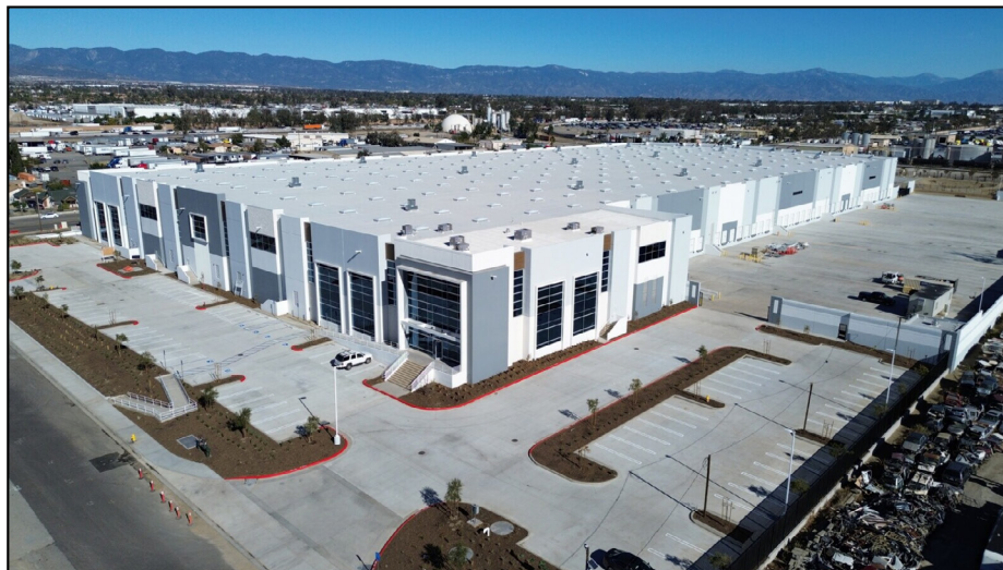
Logistics Plus 375,000 SF Warehouse in Riverside
